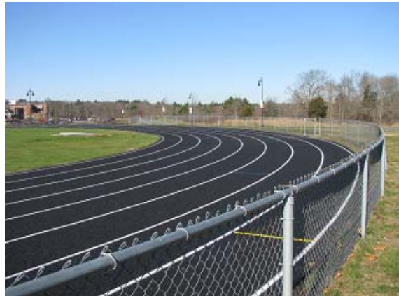
Track, Bridgewater-Raynham High School
