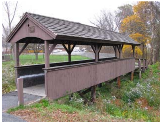
Covered bridge behind Avon Public Library
