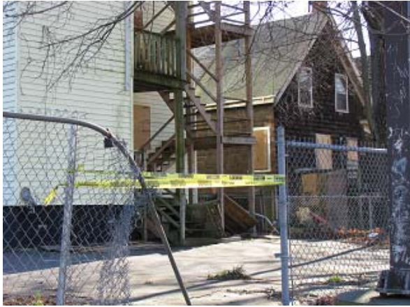
Boarded-up houses, Brockton
